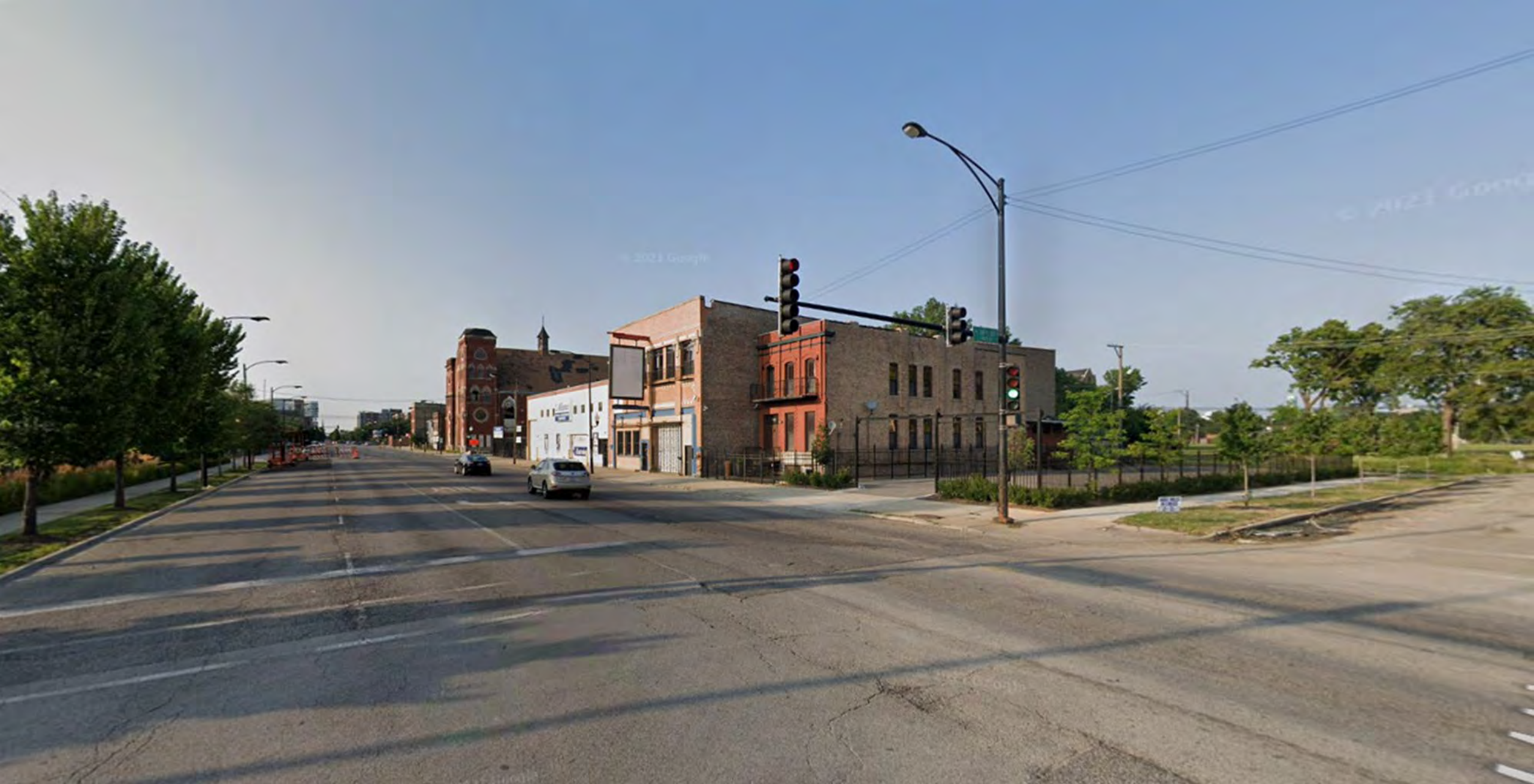
EXISTING CONDITIONS – ASHLAND/14 TH ST., LOOKING NORTH
